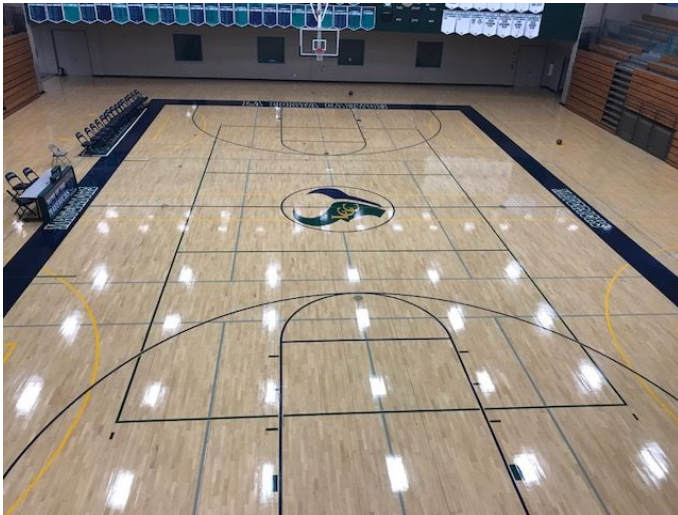
Gym Resurfacing: Completed over winter break
